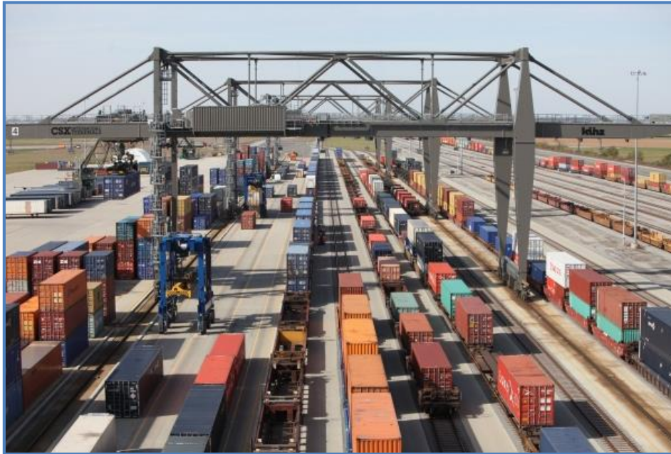
Figure 7: CSX Northwest Ohio Intermodal Terminal
